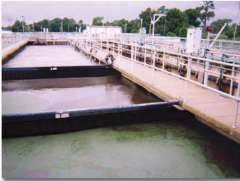
CREATE STAGED TREATMENT CELLS
