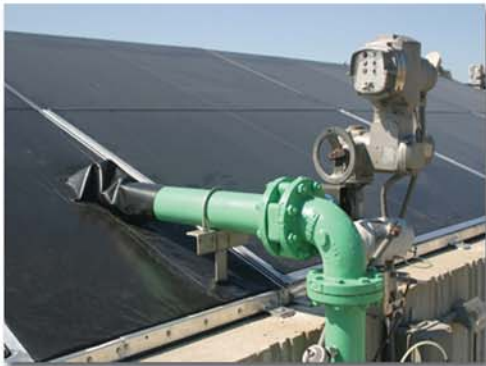
PIPE PENETRATION BOOT
